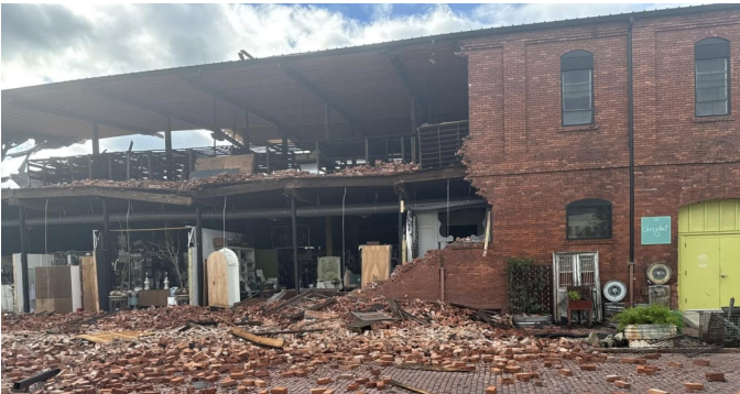
The downtown historic building housing Chez What (204 S. Ashley St.) was destroyed by Helene. photo: Chez What FaceBook
